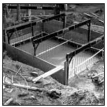
Large, three-sided configuration with hi-clearance arches and splice plates
