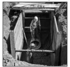
Two-sided configuration with telescoping spreaders and full length corner posts
