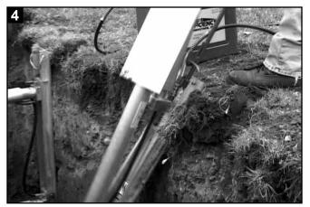
The shore will fold as it is pulled out. Remove tools, fold shore flat, and carry to the next installation spot.
