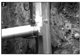
Push the tool away from you against the handle. The tool will depress the fitting and release a small amount of fluid.
