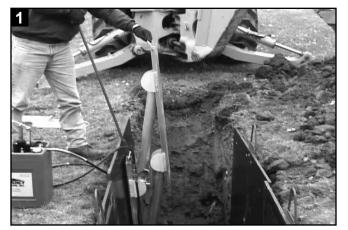
Place the shore near the trench edge in the open position with the "cylinder rail" down. Open the valve on the pump can 1/4 turn. Attach the female quick connect fitting on the pump hose to the male fitting on the top cylinder. Put the release tool through the handle on the lower rail with the hook positioned to grab the handle. Fold the shore by pulling the top rail toward you by hand. Lower the shore into the trench with hook.
