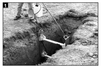
To remove the shore, place the removal tool through the handle with the hook facing the trench. Place the end of the tool over the same fitting where hose was hooked.
