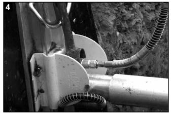
To remove the hose, place the release tool flange behind the collar of the quick disconnect fitting. The hook will be toward you. Pull the tool toward yourself, using the hook as a pivot, the hose will come off. After hose is disconnected, clip hose to the top of pump. Open valve on pump and move to the next shore.
