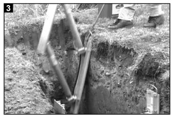
Remove from trench by pulling one side with release tool and the other side with the removal hook.
