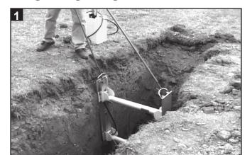
To remove the shore, place the removal tool through the handle with the hook facing the trench. Place the end of the tool over the same fitting where hose was hooked.
