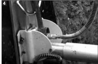
To remove the hose, place the release tool flange behind the collar of the quick disconnect fitting. The hook will be toward you. Pull the tool toward yourself, using the hook as a pivot, the hose will come off. After hose is disconnected, clip hose to the top of pump. Open valve on pump and move to the next shore.
