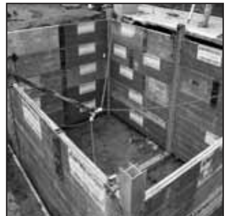
ClearSpan™ Configuration with full length corner posts
